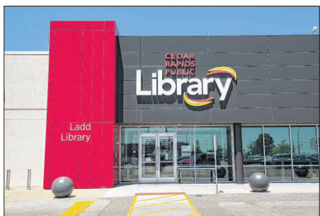
The Ladd Cedar Rapids Public Library, 3750 Williams Blvd. SW, will hold an open house Wednesday where residents can comment and ask questions about the new library and opportunity center that will be built nearby. (Nick Rohlman/The Gazette)
